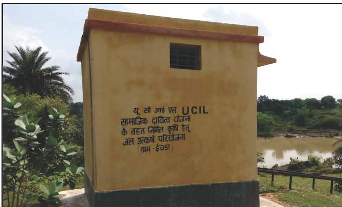
Irrigation Project at Ichra village
