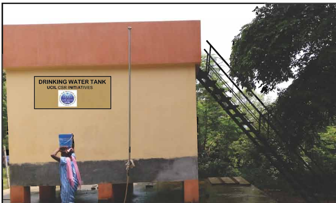
Overhead Tank at Chatikocha village
